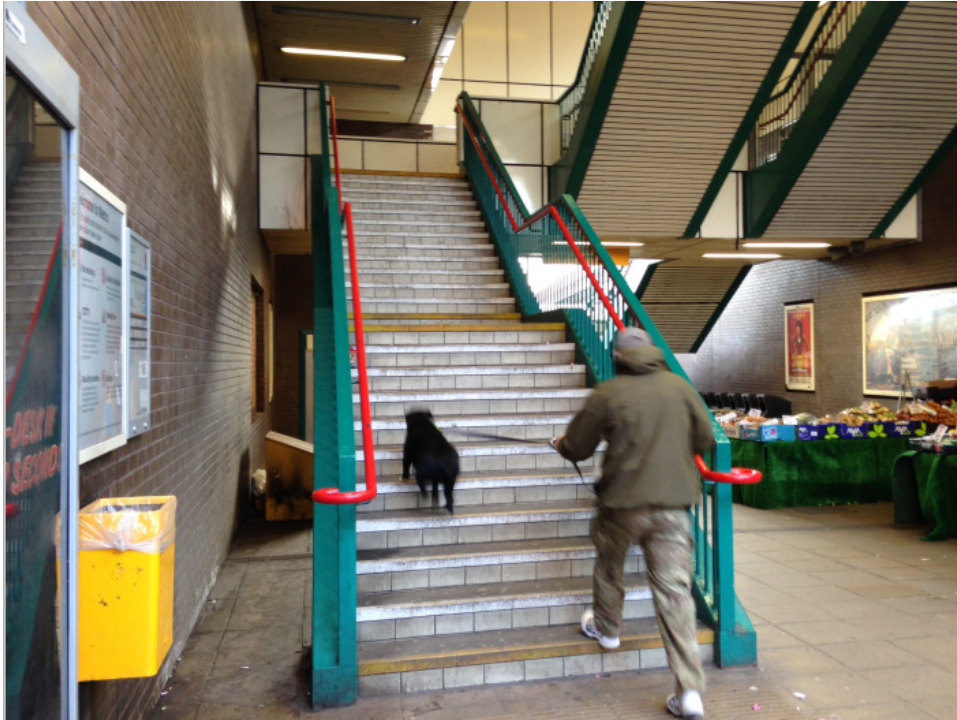
Existing Metro station entrance from King Street
