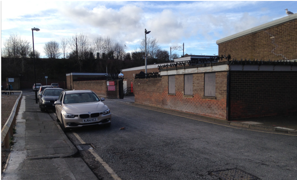
View from within the application site on Albemarle Street looking north-west at the existing Post Office building
